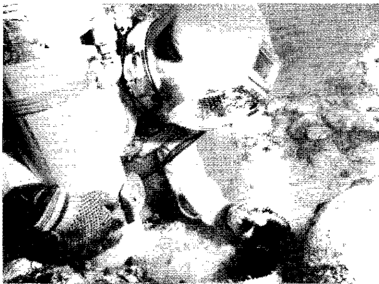
Hardhat diver excavating overburden with 150 mm airlift
