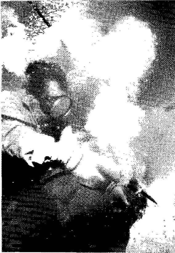
Hookah diver using pneumatic chipping hammer to remove concretion in 8 meters of water
