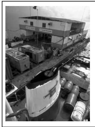
ABEX TS accommodation.
