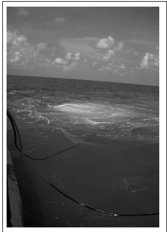
Surface signs of airlifts at work.
